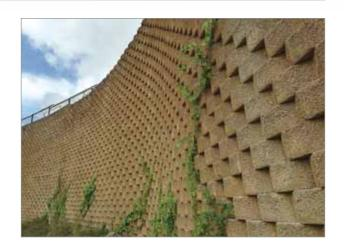
The KeySystem I, manufactured in Puerto Rico by The Paving Stone Co., a Carmelo Company, also offered Hacienda Real a dazzling wall to complement the area's natural beauty. KeySystem allows for a wide range of completed wall appearances without the cost of customization, and at 65 feet, KeySystem was the only wall system to provide the design freedom and installation ease for curves and corners.
