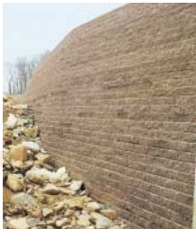
This Anchor Diamond® wall stabilized the terrain so that an emergency access road could be completed.
