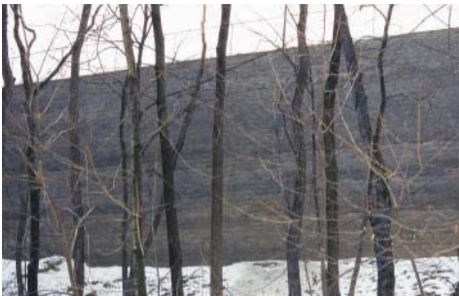
The 42-foot (12.8 meters) high Kline Plaza retaining wall rises through the trees on top of a 1.5 horizontal to 1.0 vertical slope.
