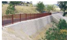
A guardrail anchored into the SRW along the Centennial Trail protects passersby from a steep embankment.
