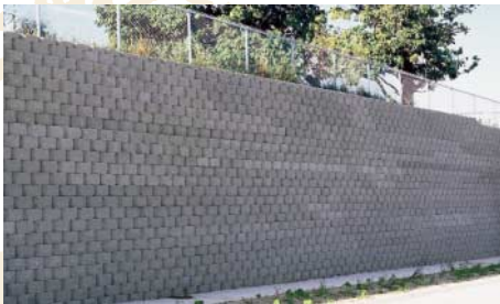
SRWs such as this one constructed using gravel backfill and pre-approved geosynthetic reinforcement can readily perform as load-bearing walls.
