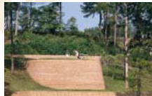
Global stability analysis helped ensure that this massive two-tiered wall on a golf course in Alabama was built with the appropriate number and lengths of geogrid.
