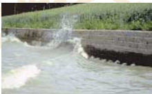
Retaining wall blocks exposed to water are particularly vulnerable to damage from subsequent freeze/thaw conditions.
