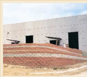
Thiele Geotech corrected a grade separation problem at the CenTech Business Park with a tiered segmental retaining wall featuring straight-faced Anchor Vertica® Pro units.
