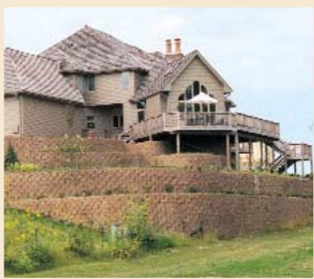
For this custom home on a golf course, Thiele Geotech designed a series of tiered walls using Anchor Vertica® units to create an attractive, economical solution to a sloping site.
