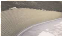
Several sections of wall surrounding the Wal-Mart parking lot were tapered to meet the changing grade of the surrounding soil.
