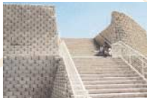
Two 50-step stairways built with Anchor Diamond® straight and beveled face units descend from the Dell Computer building facility to the parking lots.
